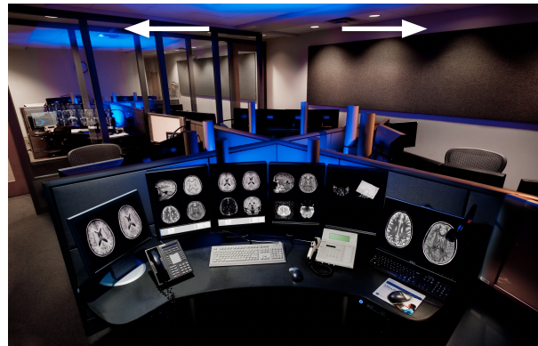
Sound absorbing panels; Acoustical separation using glazing
